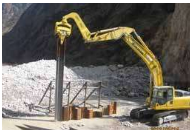
Photo 1: Installation of Sheet Piles
