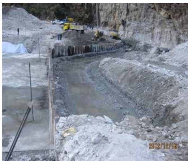
Photo 6: Established JGC wall and Installed Sheet piles (View:: Left to Right)
